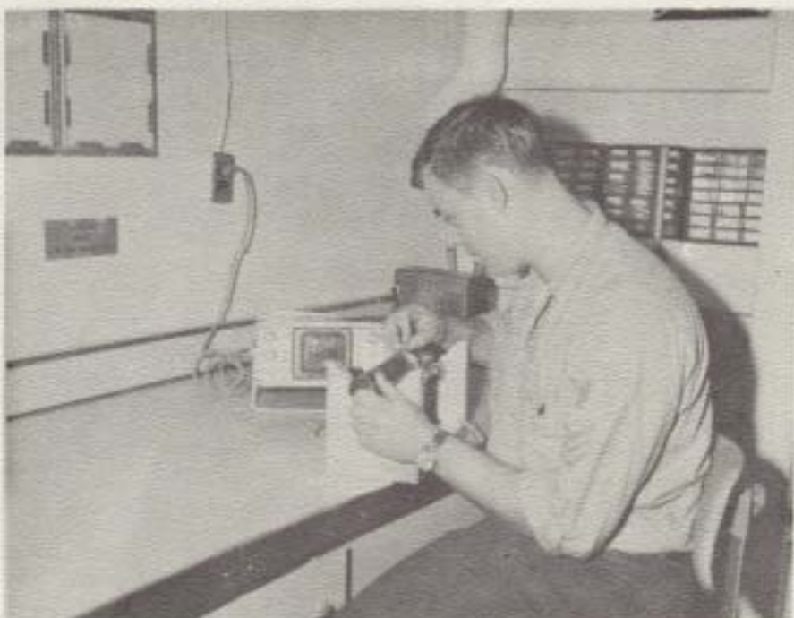
SF1 R. A. ANDERSON performing an ultrasonic soundwave inspection of a silver brazed joint non-ferrous pipe.
